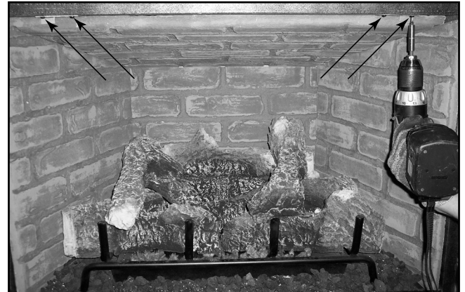
Figure 7.19 Remove Refractory Retainers
